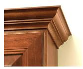
**Crown Moulding** - goes on top of the cabinet. May or may not connect cabinet with the ceiling.
